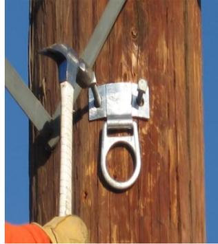
Use 2 factory supplied fasteners supplied with the Rescue MUTT
