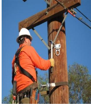
Start the ½” x 5” Kortik Lag Screw bolts using a hammer
