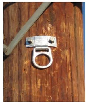
Make sure that both lag Screw Bolts are in all the way
